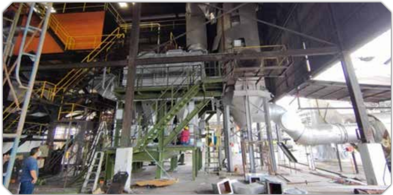
Figure: Installation of Vorcep Air Pollution Control System in SAI's oleochemical plant in Kapar, Selangor.
