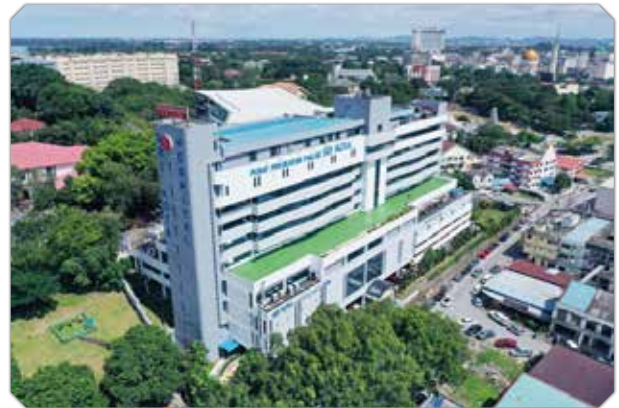
Figure: View of Sri Kota from above.
