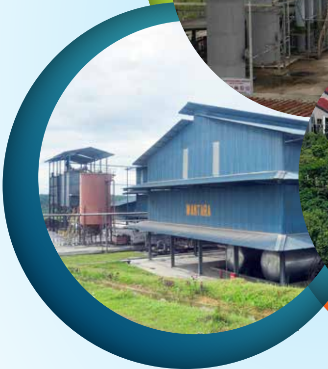
Milling & Estate Segment
